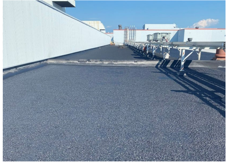
Elastomeric Membrane – Ertech 3035 prior to roofing granule application
