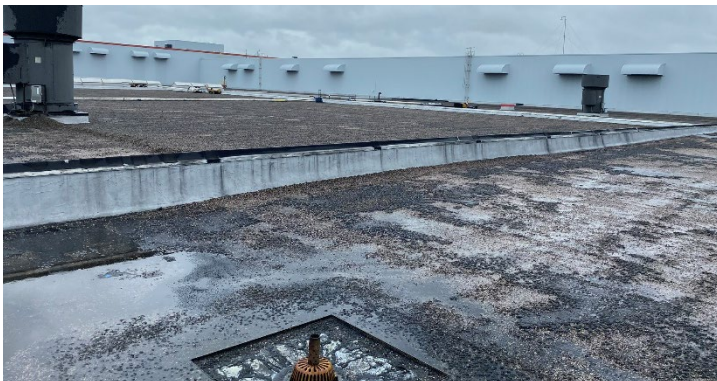
Before restoration – Aged modified bitumen roof with multiple penetrations
