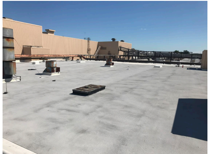
Finished Restoration – White roofing granules over Ertech 3036 adhesive
